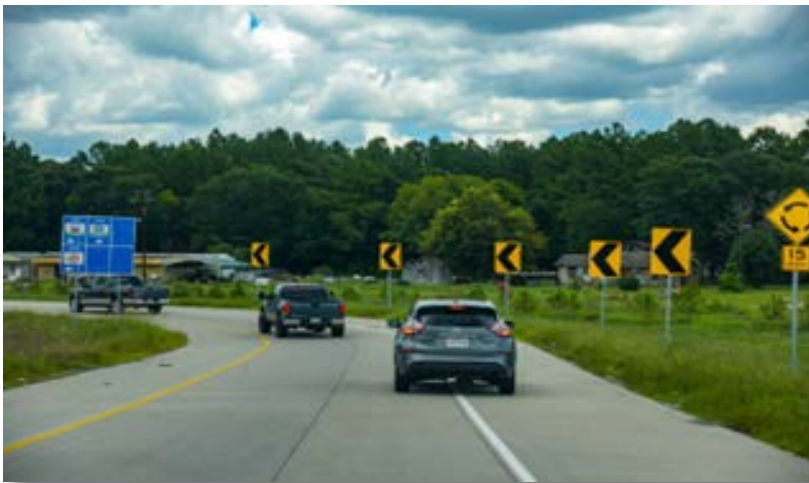
Vehicles navigate a curved highway ramp marked with bright directional signs. (source TTI)
