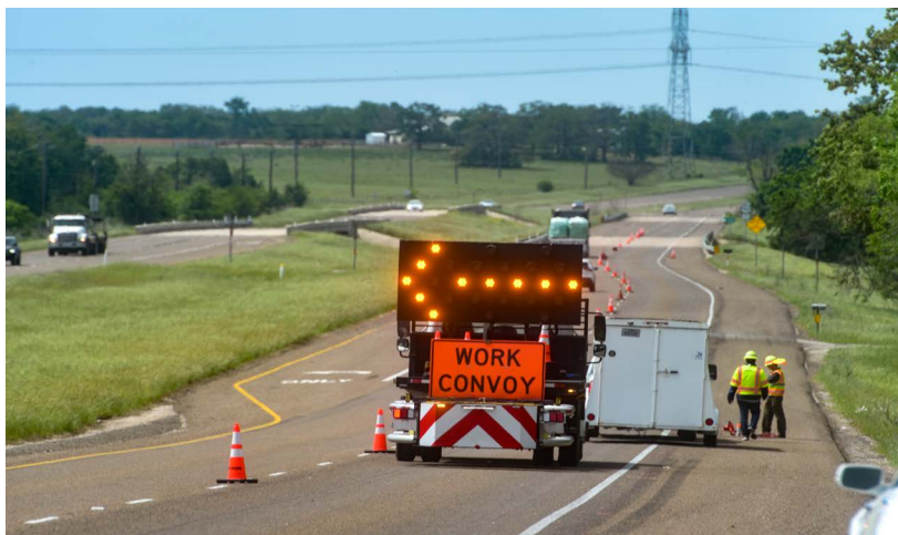
Highway crew manages work zone with cones and convoy vehicle guiding traffic. (source TTI)
